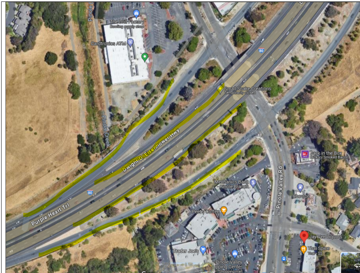
I-80 at Pinole Valley Road
