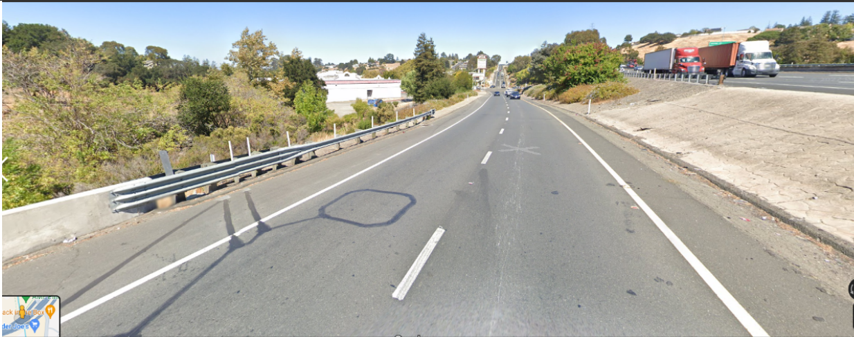
West-bound on-ramp at creek over crossing (note the guard rail that allows trash to flow freely into creek)
