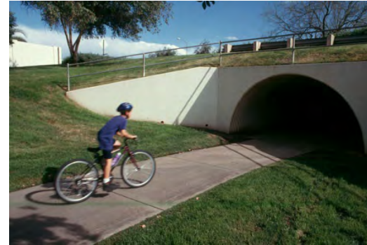
Source: www.pedbikeimages.org / Dan Burden
