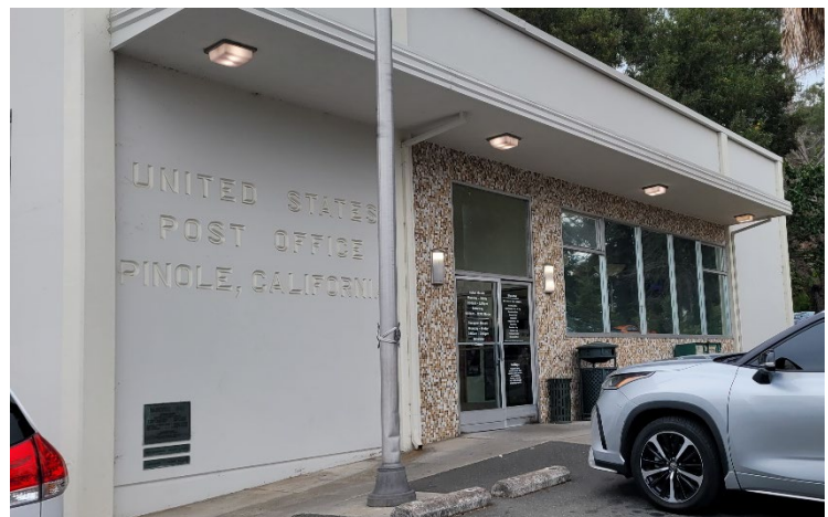
Post Office and Exterior Lighting
