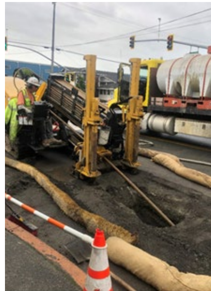
Figure 21 Directional Bore
