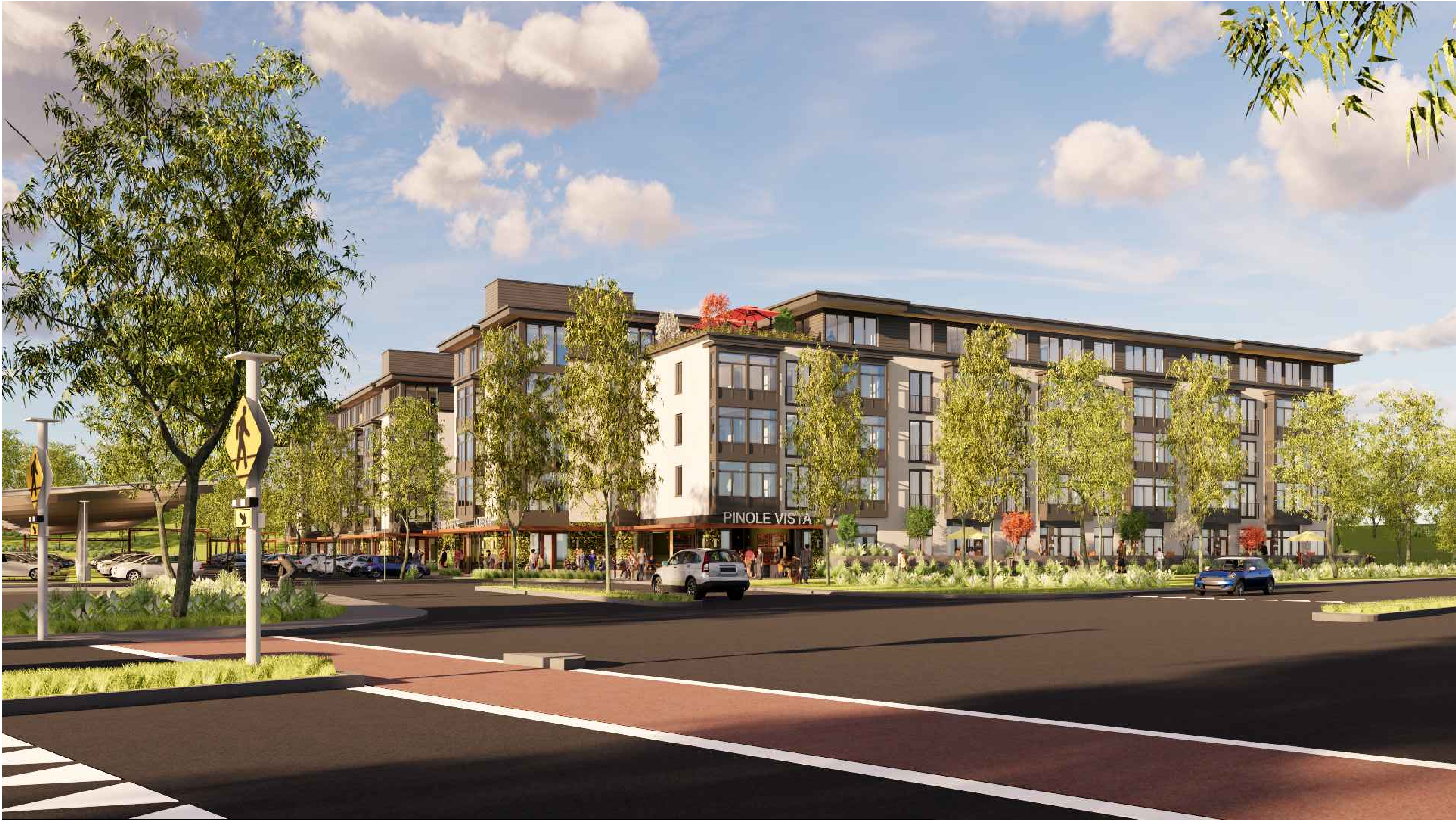
1 VIEW OF MAIN PROJECT ENTRY
