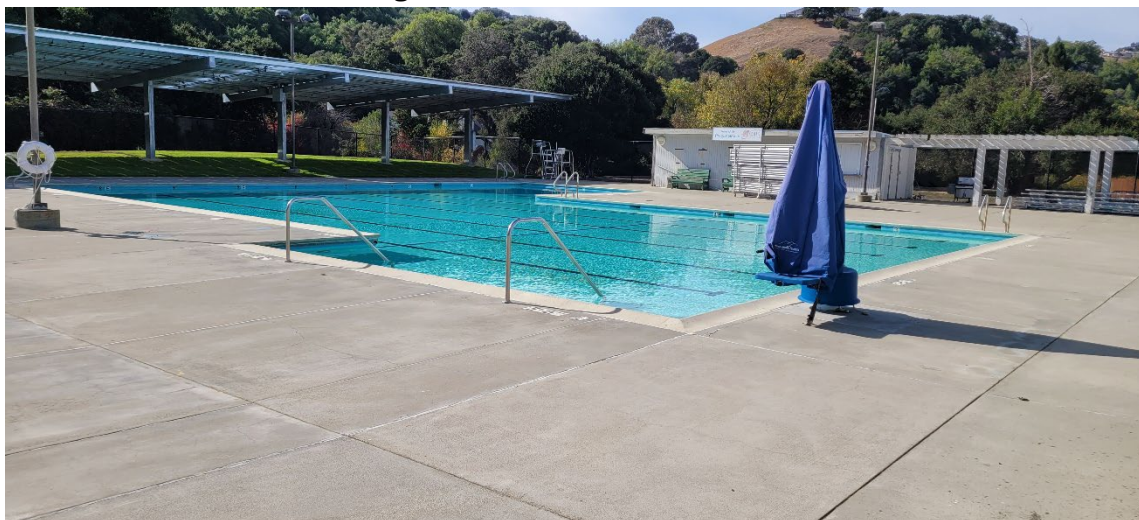
Figure C.22 Uncovered Main Pool
