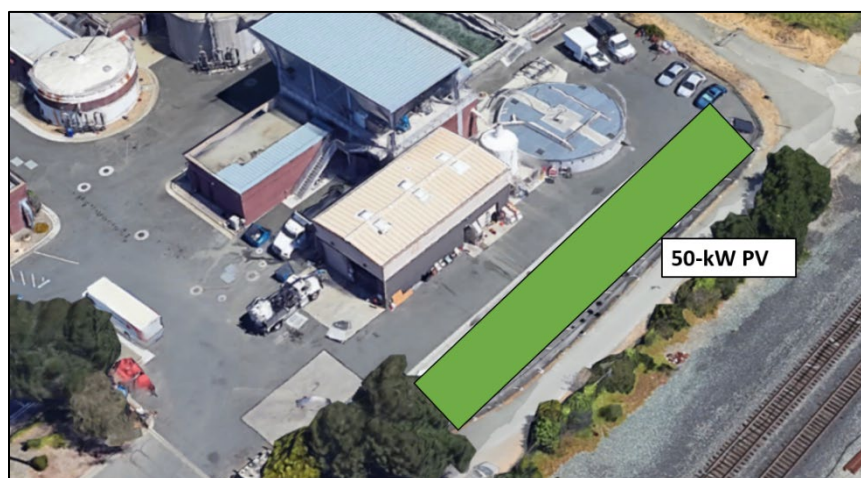
Figure C.11 Carport PV Location
