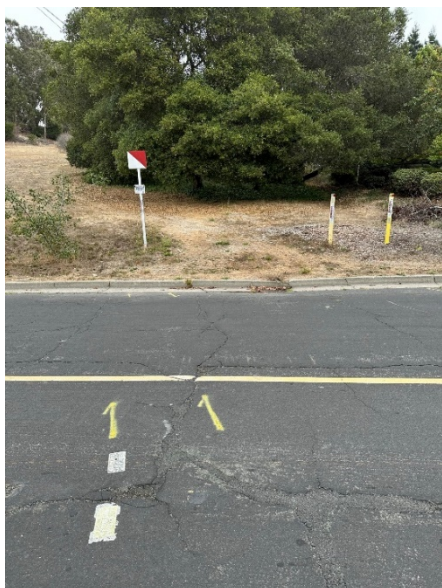
Figure 2 Petroleum line crossing Pinon
