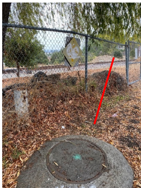
Figure 3. Sewer crossing BSNF railroad
