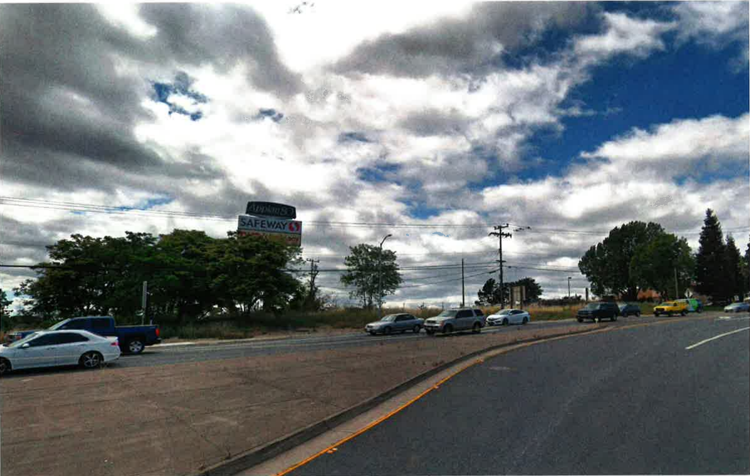
INTERSTATE 80 AND APIAN WAY INTERCHANGE LOOKING NORTHWEST VIEW OF EXISTING CONDITIONS
