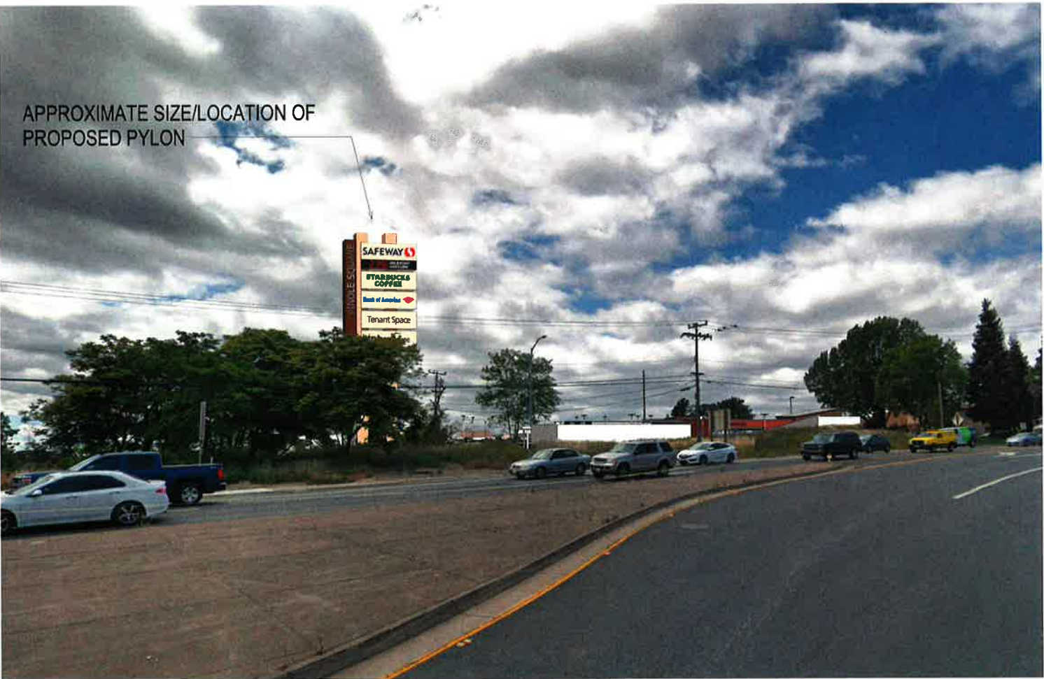
INTERSTATE 80 AND APIAN WAY INTERCHANGE LOOKING NORTHWEST VIEW OF THE PROPOSED PROJECT
