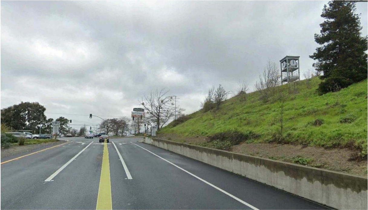
180 AND APPIAN WAY INTERCHANGE WESTBOUND OFF RAMP
