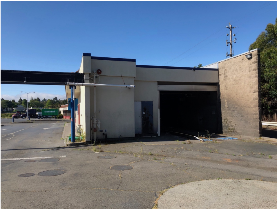
Photograph 6. Former car wash structure.
