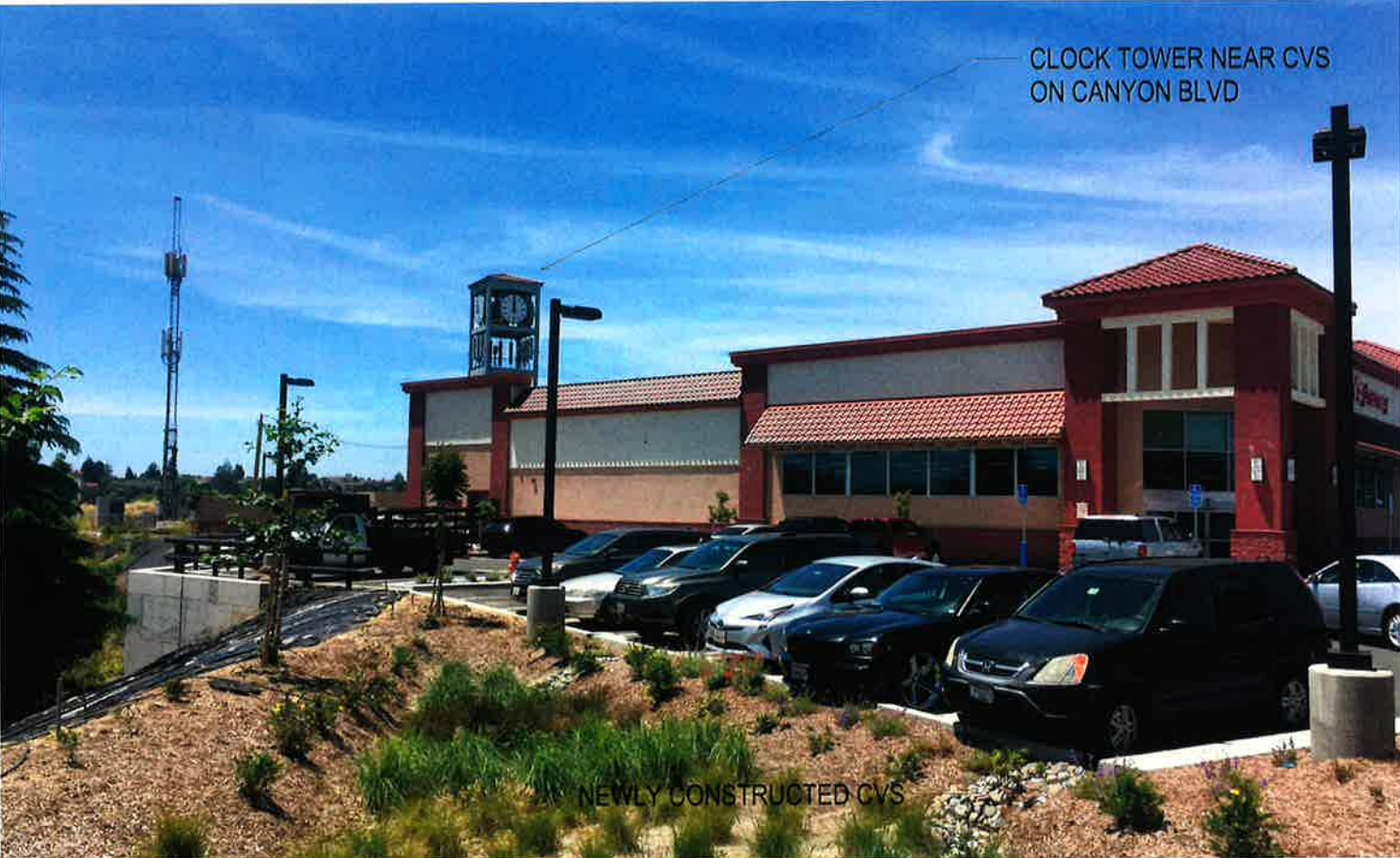
VIEW FROM ACROSS HIGHWAY OF EXISTING CONDITIONS
