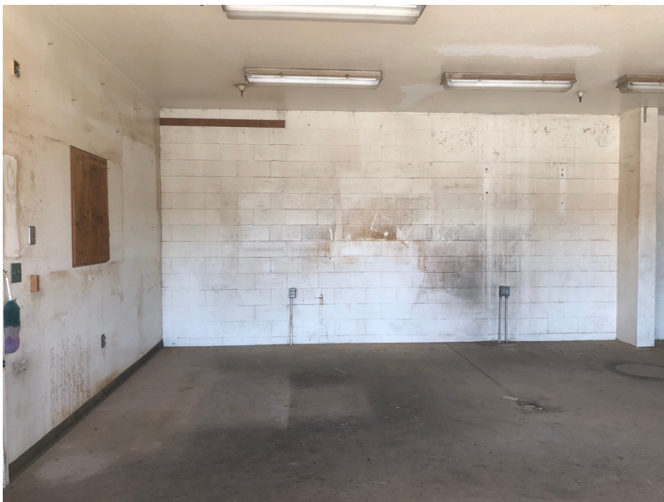
Photograph 10. Interior of former Antiques Restoration.
