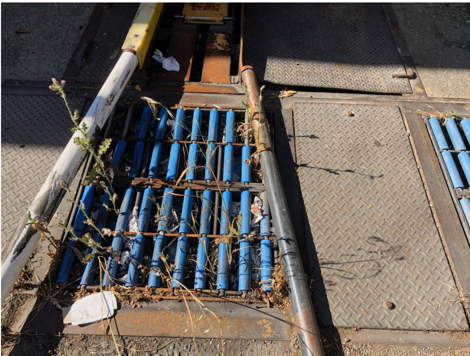
Photograph 8. Drains associated with former car wash.
