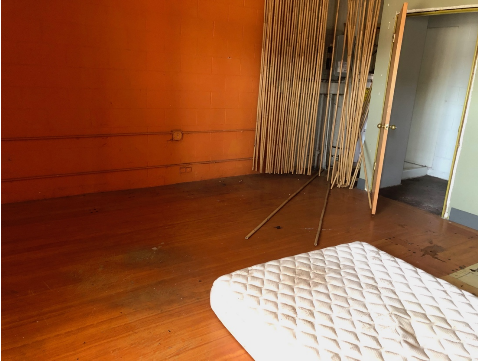
Photograph 11. Additional room inside former Antiques Restoration.
