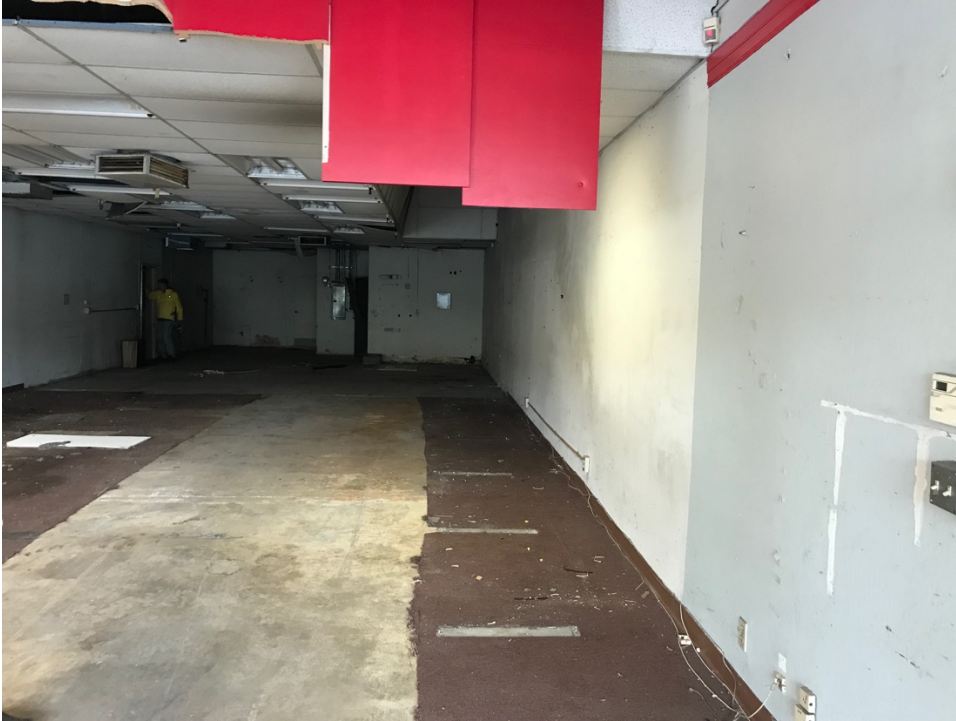
Photograph 31. Interior of former Four Mile Cleaners.
