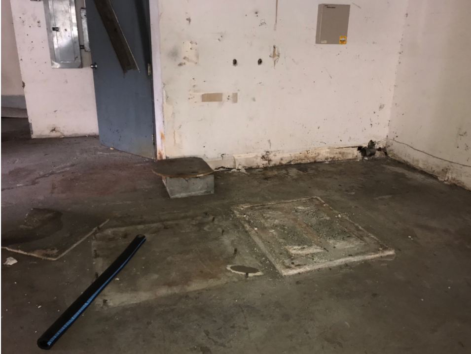
Photograph 34. Previous location of dry cleaning equipment.
