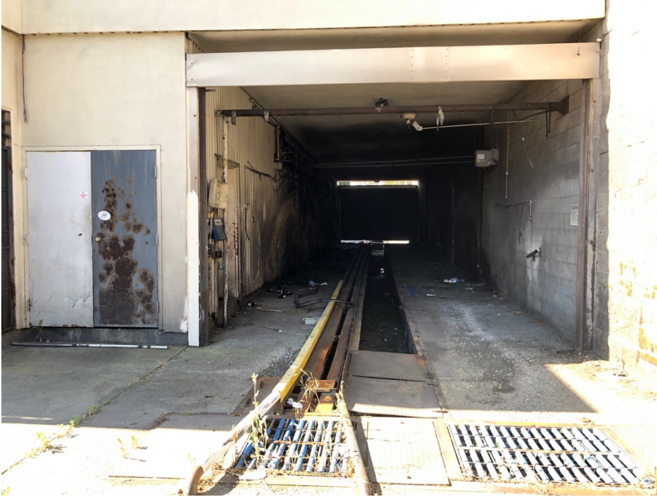
Photograph 7. Car wash automatic wash bay.
