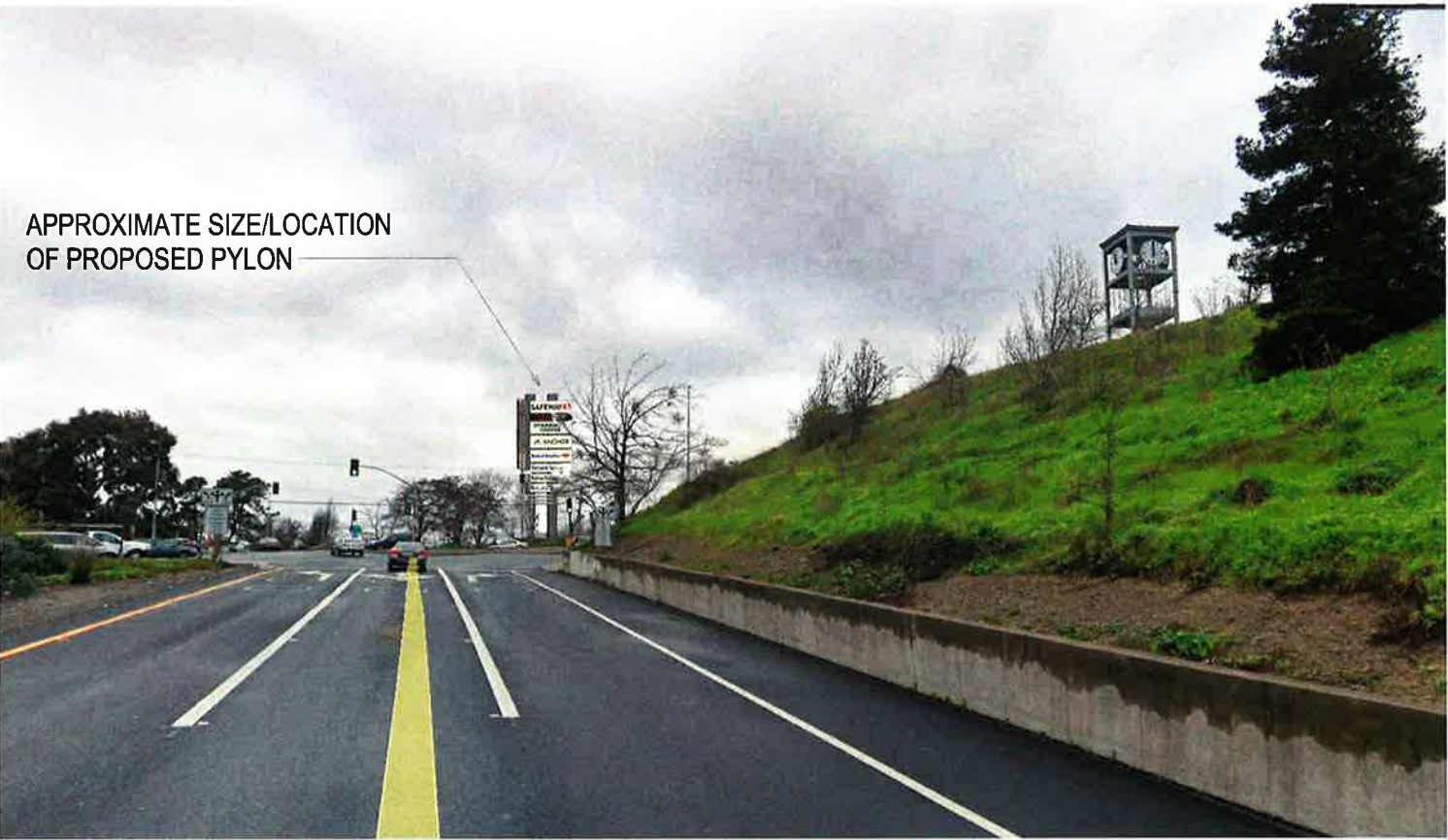
180 AND APPIAN WAY INTERCHANGE WESTBOUND OFF RAMP
