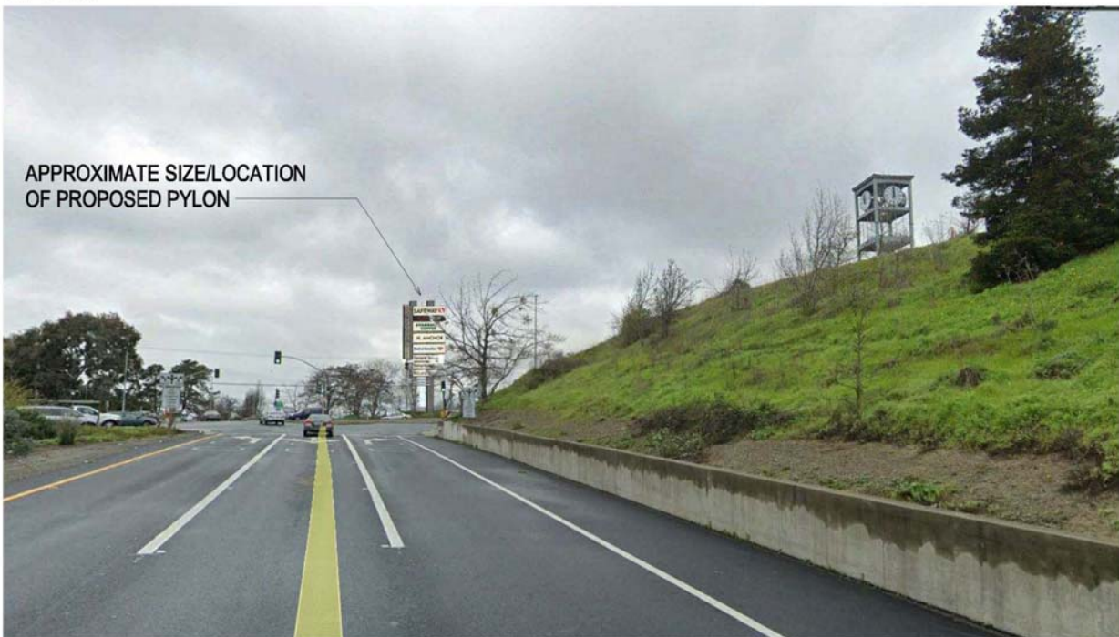
180 AND APPIAN WAY INTERCHANGE WESTBOUND OFF RAMP
