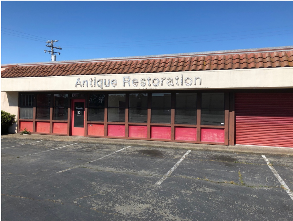
Photograph 9. Former Antiques Restoration structure.
