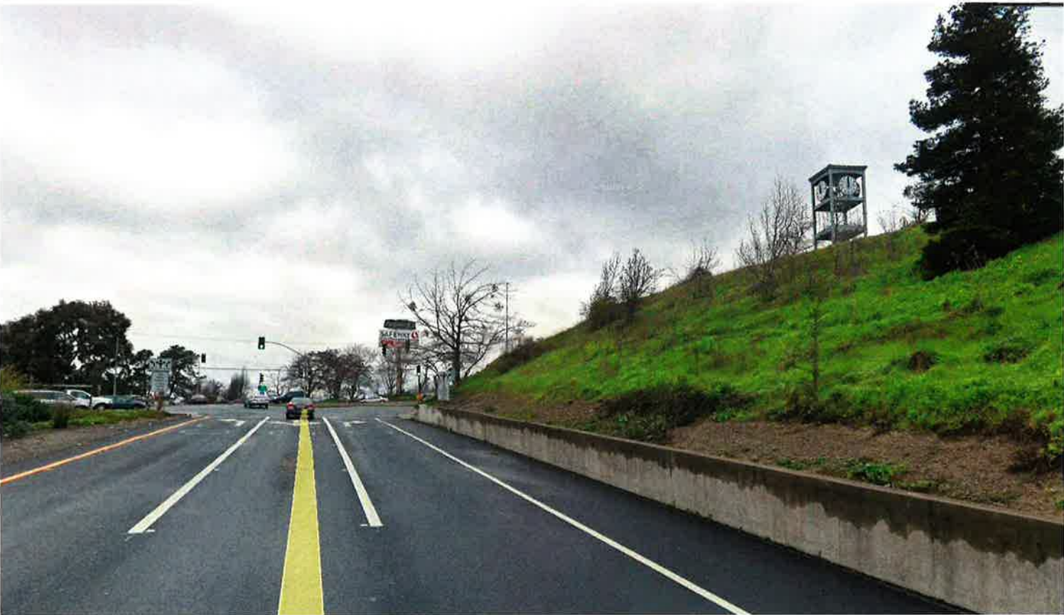
180 AND APPIAN WAY INTERCHANGE WESTBOUND OFF RAMP
