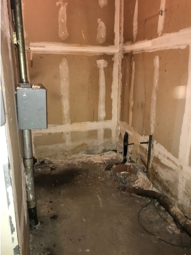
Photograph 33. Previous location of dry cleaning equipment.
