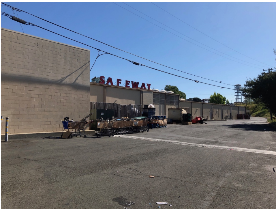
Photograph 19. Rear of Safeway store.
