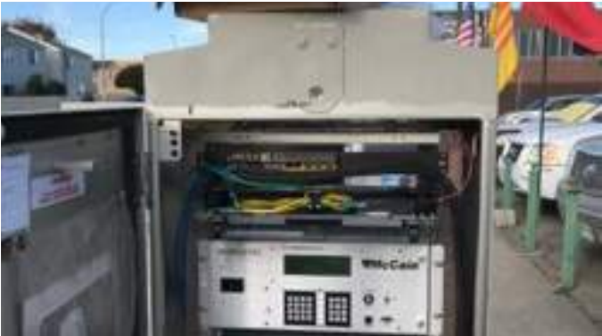
ITS backed by a fiber optic network is fundable by both State and Federal grants. Designed properly, these systems can also serve as municipal networks. Picture here is the City of Richmond municipal network, which also interconnects 23rd and 22nd Street corridors. CCTA has a plan to complete a traffic signal interconnect project in Contra Costa County, which could be leveraged to support municipal broadband services.
