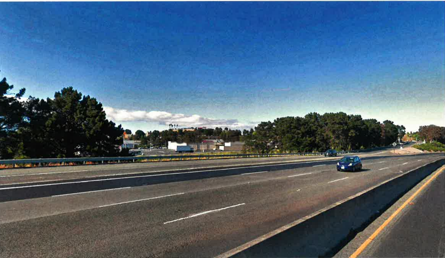
INTERSTATE 80 EASTBOUND VIEW OF THE EXISTING CONDITIONS
