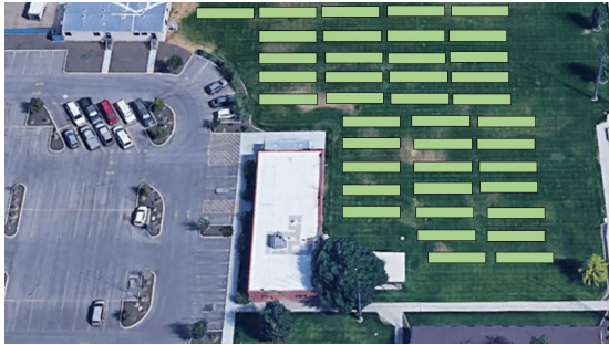
1,560 panels, 600-kW system
