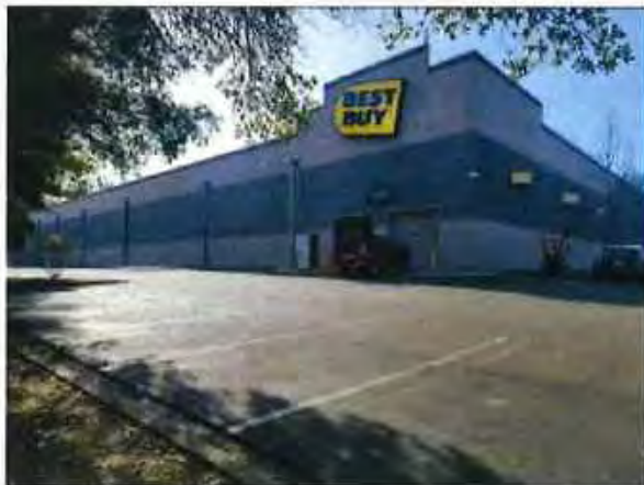
17. View of the commercial land use observed adjacent to the west of the subject property.
