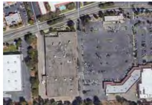
Figure 2: Existing Site Conditions
