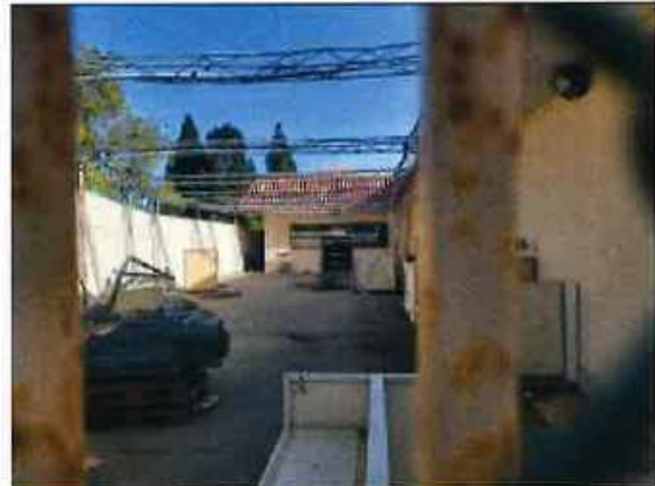
12. View of the northwest side of the building in the subject property.
