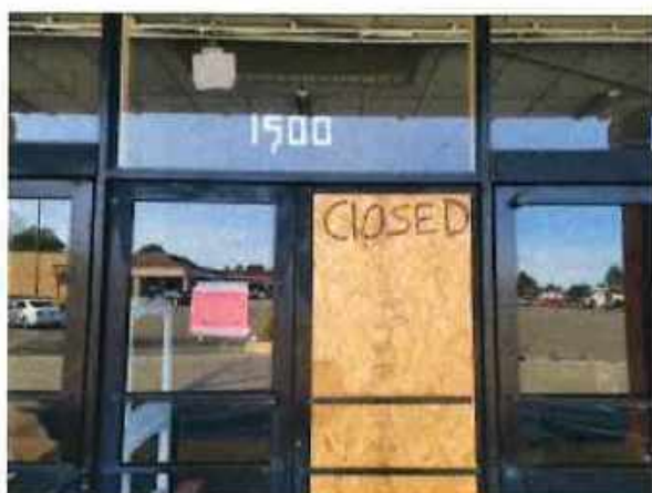
3. View of the subject property building entrance.
