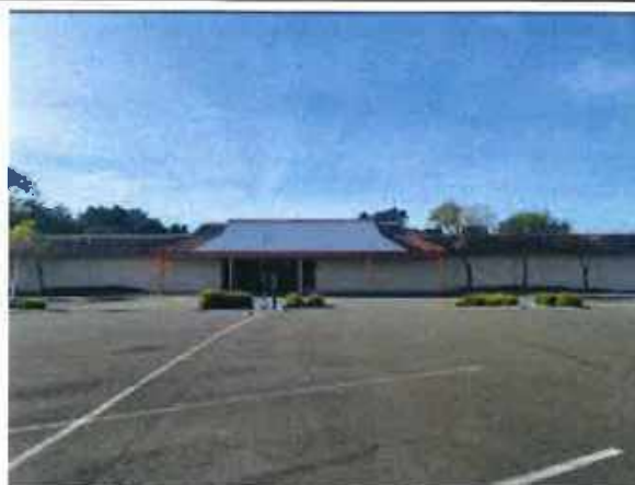
2. East view of the parking lot and currently vacant building in the subject property.
