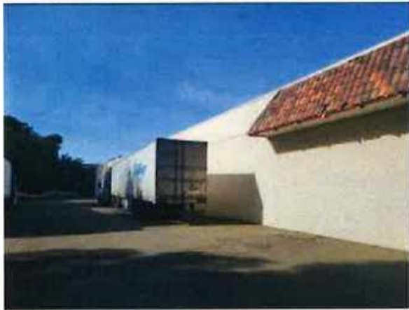
7. South view of the building on the subject property.
