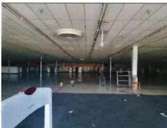
6. View of the internal condition and observed through a glass door on the central portion of the building in the subject property.
