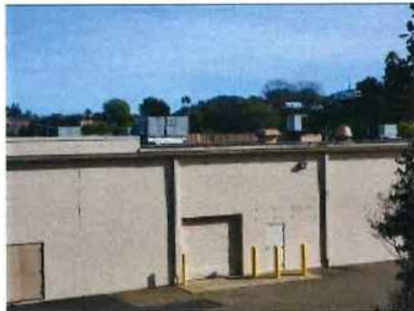
11. West view of the building in the subject property.
