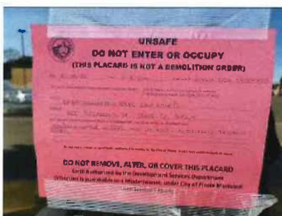
4. View of a City of Pinole ordinance restricting access to the building interior.
