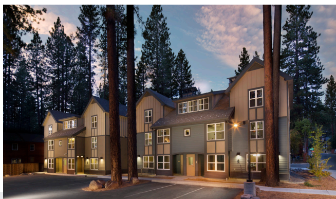
KINGS BEACH FAMILY HOUSING Kings Beach, CA – 2012
