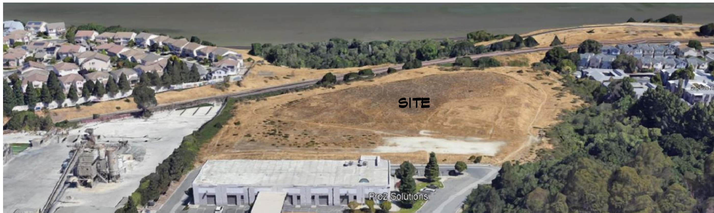
5 SOUTH AERIAL VIEW
