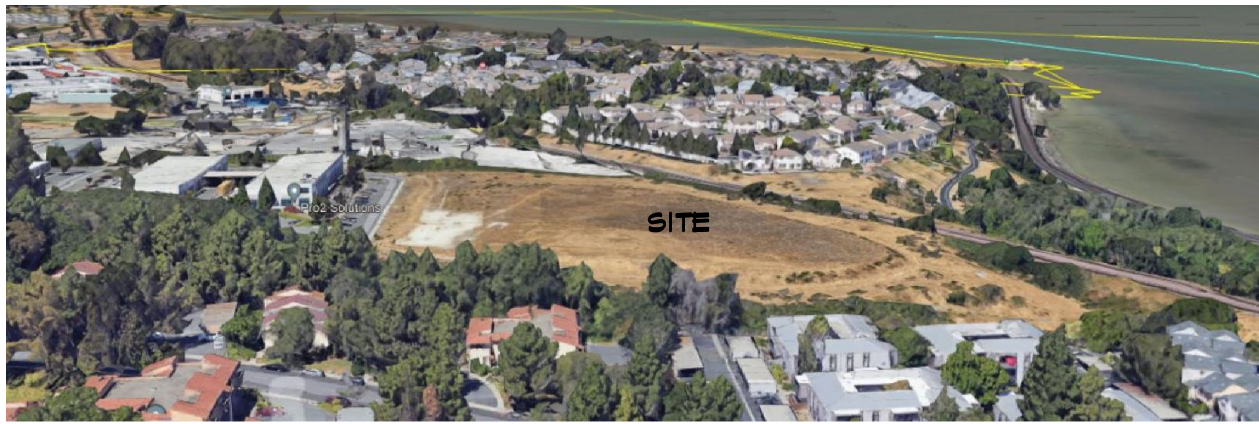
2 EAST AERIAL VIEW
