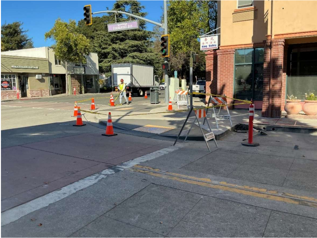
At Intersection of San Pablo Avenue/Fernandez Avenue
